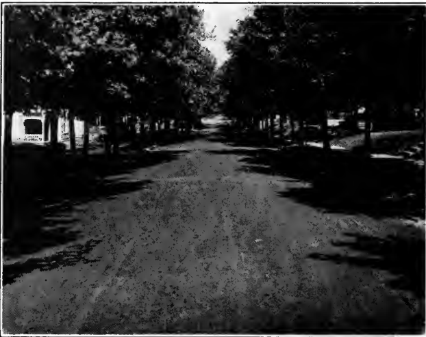
NORTH 21ST STREET, A BITUMINOUS GRAVEL ROAD IN RICHMOND, IND.
